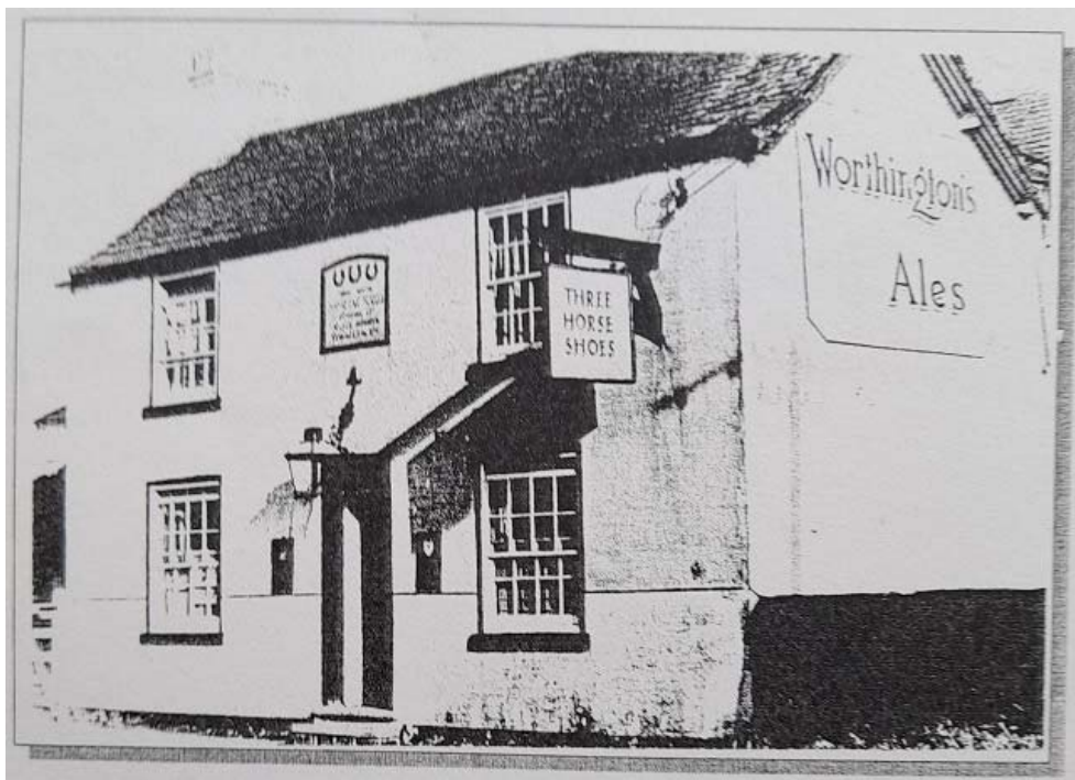
The Three Horse Shoes - demolished 1966
