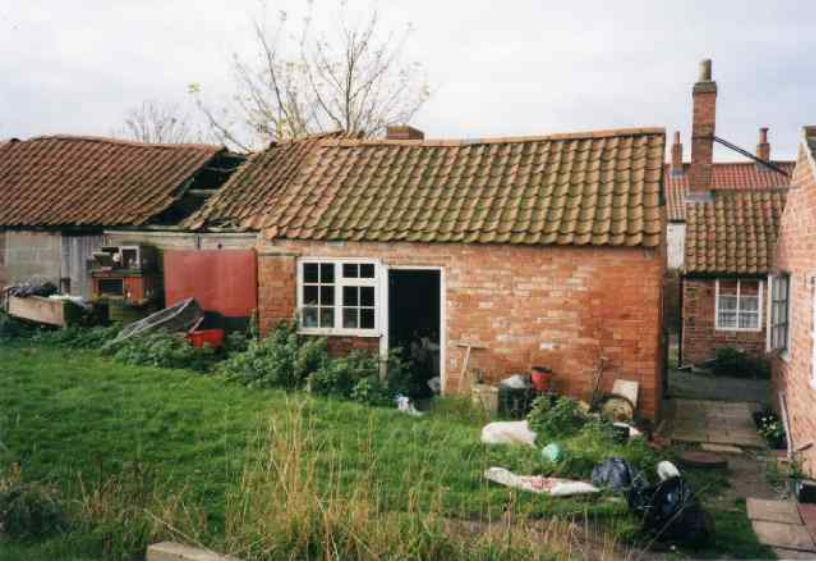
Remains of the joinery workshop (far left) behind the large grey door.
